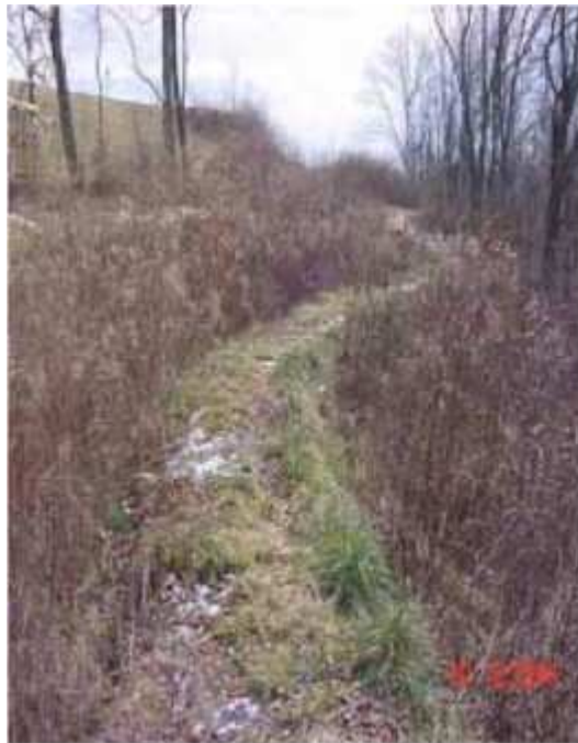
Figure 9-33. This grassy path is an embankment, or berm, creating depressions for recharge trenches located to the left of the path.
