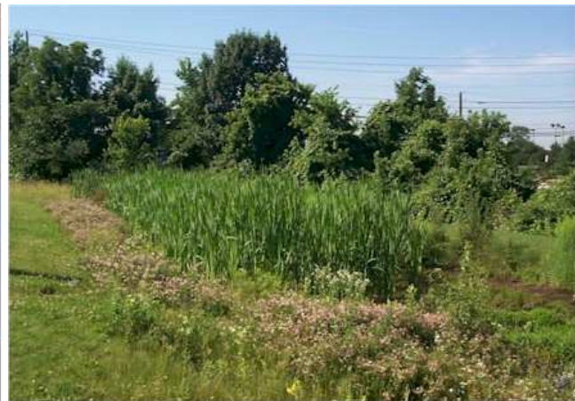
Figure 9-17. Vegetated infiltration filters.
