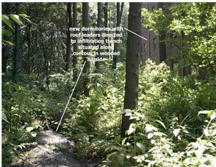
Figure 9-27. Level spreader pipe/infiltration trench in woods.
