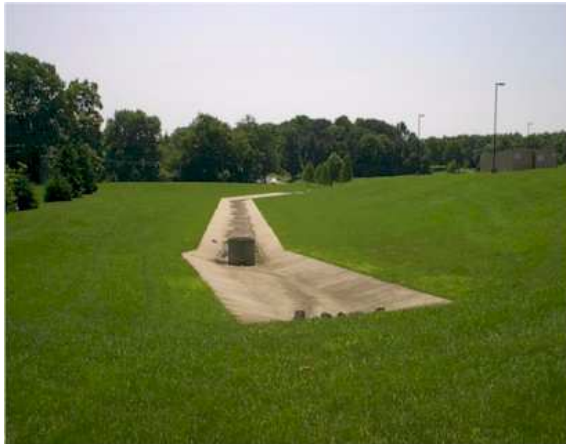
Figure 9-25. Existing sinkhole-plagued detention basin.
