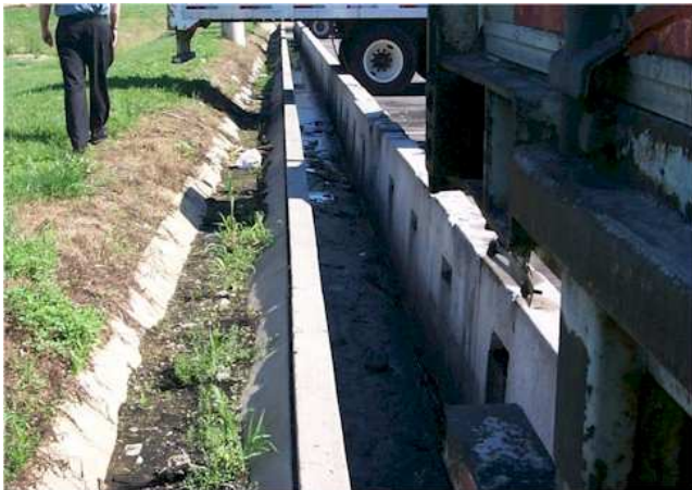
Figure 9-16. Perimeter trench drain.
